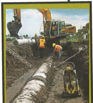
I-95 Brevard County: Installation of 30 inch outfall to control structure in Pond 15
