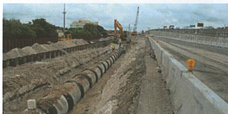
42 inch pipe installation
