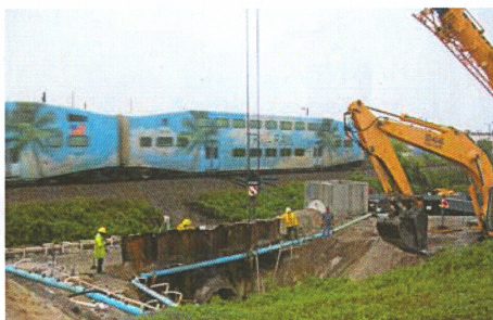
NW 21st Avenue Broward County: 72 inch bore pit beneath the CSX railroad ROW
