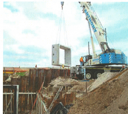
Lakeside Ranch: Installation of pre-cast 16 foot x 12 foot box culvert for Dickerson Florida Inc. and the South Florida Water Management District
