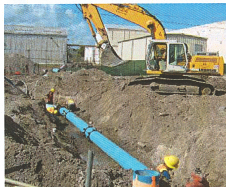
Installation of 16 inch water main
