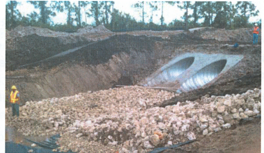
C-44 Reservoir/C-133 Canal: Preparation and final 84 inch culvert construction for Hardrives Inc. and the South Florida Water Management District
