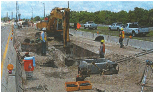
Dixie Fly-over: Installation of 36 inch French Drain for Cone & Graham Inc. and the FDOT
