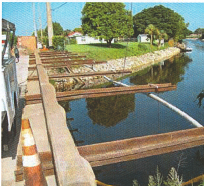
Juanita Avenue Bridge/ St. Lucie County: Temporary relocation of 1800 pair cable for AT&T
