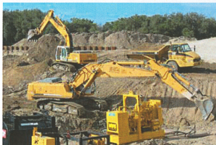
Excavation and preparation for FC-1 control structure
