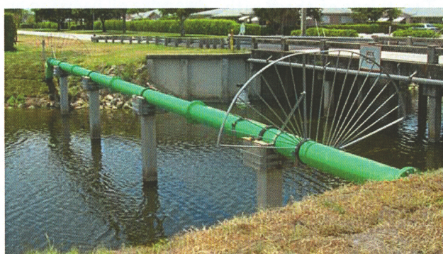
LS 50 E-4 Canal Crossing: Replacement of existing 12 inch force main (above left) then final product with fan guards fabricated by our shop (above right)
