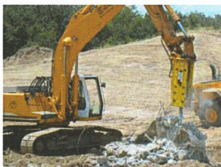
Final demolition of existing concrete structure prior to offsite removal
