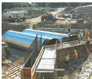
108 inch diameter culvert supplied by our longtime Lantana neighbors at Con-tech Construction Products
