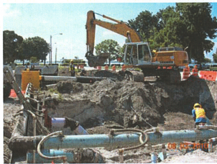
Wellpoint dewatering to install pressure piping as a result of high water table
