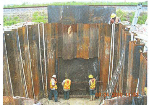
NW 21st Avenue: Preparation of bore pit beneath the CSX railroad right of way for Ranger Construction Industries and Broward County
