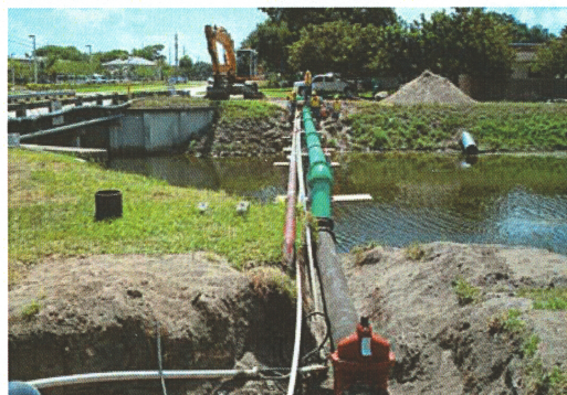
LS 50 E-4 Canal Crossing: Replacement of existing 12 inch force main (above left) then final product with fan guards fabricated by our shop (above right)
