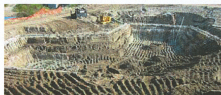
Final "footprint" being excavated after successful dewatering operation
