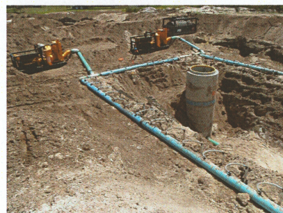
Properly installed dewatering system
