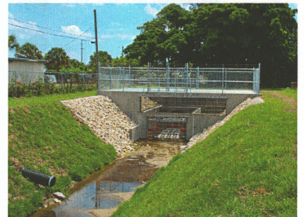
RC-4 Canal Water Quality Improvement (above): Preparing the slopes for rubble and after installation of pollution control bafflebox for the City of Riviera Beach. The extensive grating system was fabricated "in house" by our shop personnel.
