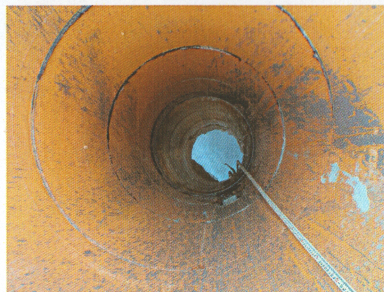
Looking down into the Aggru-Lined lift station which is 8 feet in diameter and 25 feet deep installed in a 25 foot water draw down
