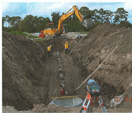
18 inch RCP drainage installation
