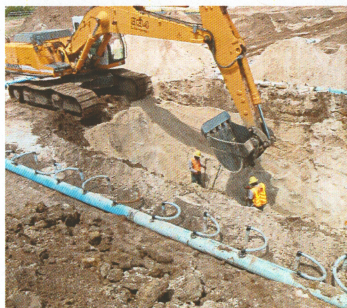
Laying 8 inch gravity sewer
