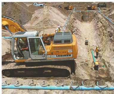
Installation of 8 inch gravity sewer
