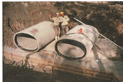
1992: One of our first City of Port St. Lucie annual culvert replacement contracts. Bobby Hall and Cleveland Evans install large diameter elliptical pipe across Airoso Boulevard.
