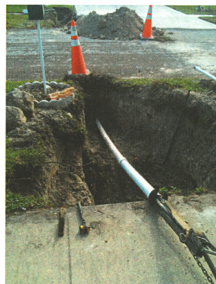
South County Service Replacement: 3" PVC casing pipe being pulled back through trenchless hole for the Palm Beach County Utilities Department.
