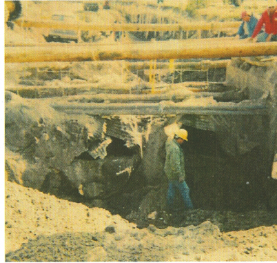
1991: Virginia Avenue/SR 70 was our first project in the Ft. Pierce area, constructed for Ft. Pierce Contracting and the FDOT. AT&T ducts, forcemain, watermain, and gasmain were supported to remove existing pipe and replace with a new 84 inch concrete pipe. Current Mainline Foreman Jeff Brady was pipelayer on the crew.
