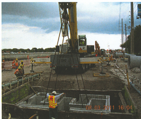
Odilon Hernandez and crew setting a 17'x12' weir control structure.
