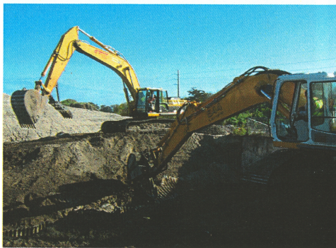
Culvert 14: (Left) Pipe culvert demolition for the US Army Corps of Engineers, working in partnership with prime contractor Optimum Services. (Center): Headwall demolition in preparation to dewater to required elevation. (Right): Excavation and dewatering prior to levee reconstruction.
