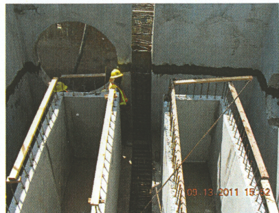
Due to its size, Odilon Hernandez and crew had to field assemble this weir control structure that was precast by Concrete Products of the Palm Beaches.
