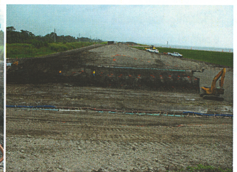
Culvert 14: (Left) Pipe culvert demolition for the US Army Corps of Engineers, working in partnership with prime contractor Optimum Services. (Center): Headwall demolition in preparation to dewater to required elevation. (Right): Excavation and dewatering prior to levee reconstruction.
