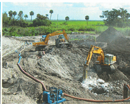
Culvert 14: (Left) Pipe culvert demolition for the US Army Corps of Engineers, working in partnership with prime contractor Optimum Services. (Center): Headwall demolition in preparation to dewater to required elevation. (Right): Excavation and dewatering prior to levee reconstruction.
