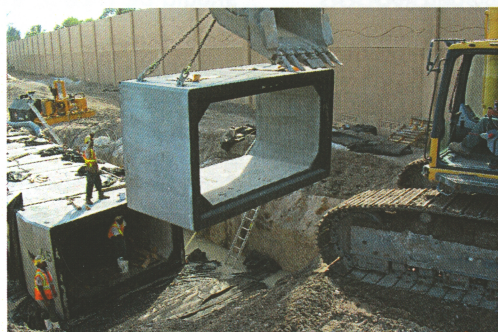
12'x6' box culvert installation in Segment E.
