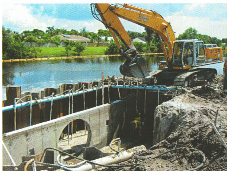
Jeff Brady and crew installing 72 inch endwall along the New River Canal.
