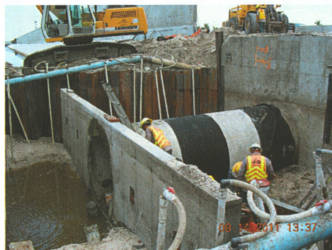
Jeff Brady and crew completing 72 inch wall installation.
