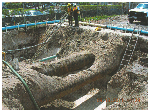
Chescal Ceance and crew installing large structure while working around multiple existing utilities.
