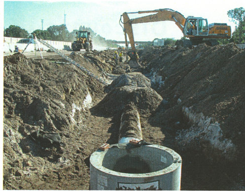
I-95 Design Build for Hubbard Construction Company: Installation and backfill of 24 inch PVC drainage piping on the 14 mile interstate widening.
