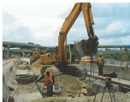
SR 112: Odi Hernandez and crew installing Inlet in tight quarters in the median in Miami for Condotte America.
