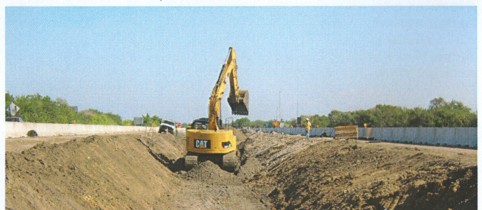
Dave Richards's crew installing 36 inch RCP north of SR50.
