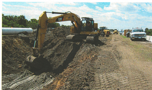
Dave Richards's crew continuing benching the day after the photo to left, managing the constantly changing conditions.
