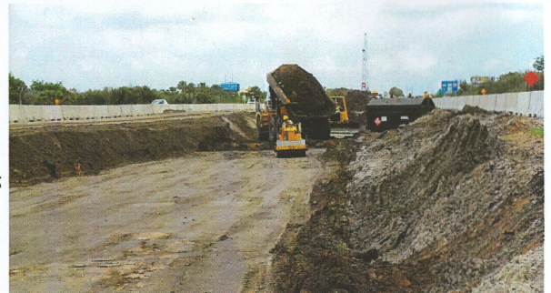
Completing backfilling over 36 inch PVC south of SR 50.
