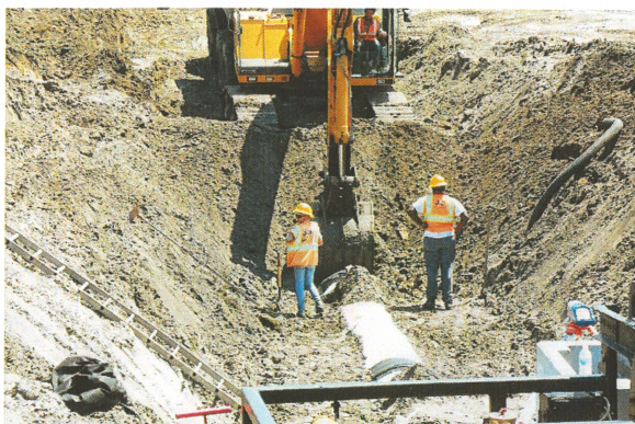
Installation of 36 inch PVC by Sean Delahunty, Jodie Kirk, and Willie Woolridge.
