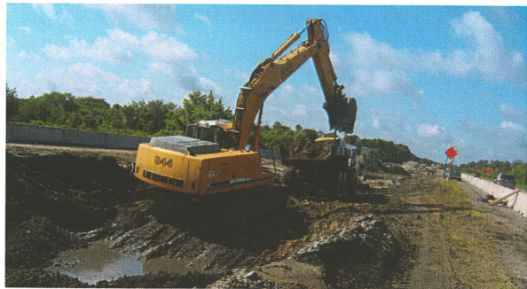
Dave Richards's crew benching down for 36 inch PVC installation south of SR 50.
