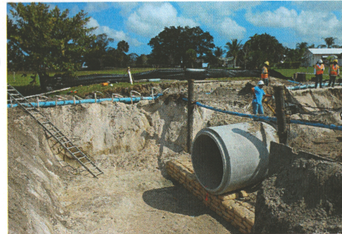
Installing 60 inch RCP with footer made of riprap bags while inspector observes.
