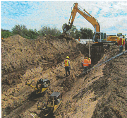
David Reid's crew of Mateo Torres Mendez, Andres Pascual, and Manuel Hernandez installing 30 inch PVC pipe down the median.
