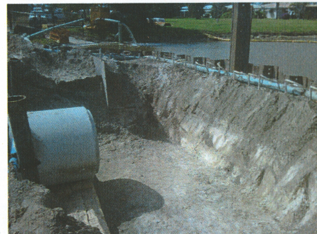
Installation of the north portion of a new culvert at Mainland's.
