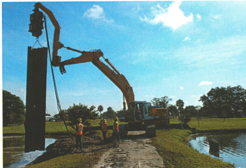
Chescal Ceance's crew sheeting prior to installation of 60 inch crossing.
