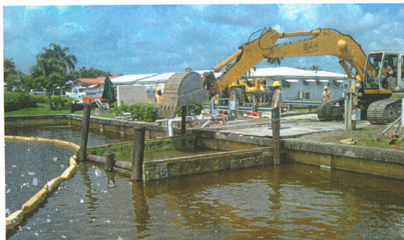
Prior to dewatering the south portion of a new 60 inch culvert at NW 46th Street.
