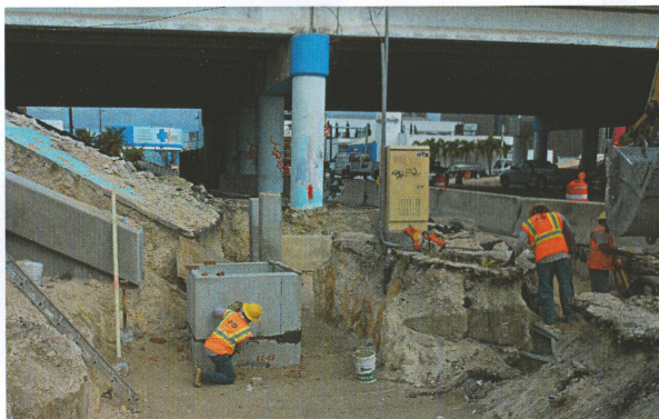
(Right) Port of Palm Beach Slip 3: Norm Weaver and crew installing 48 inch RCP for Rosso Paving & Drainage.
