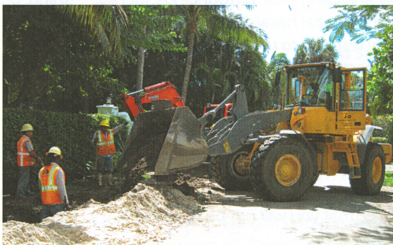
Palm Trail Area Drainage Improvements: Odi Hernandez's crew backfilling after installation of 12 inch HDPE in a community for Rosso Paving & Drainage.
