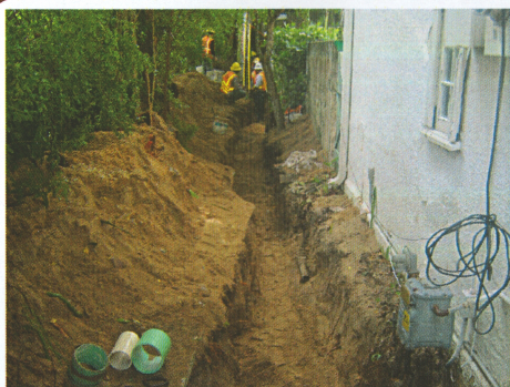
Town of Palm Beach Sewer/Storm Rehabilitation: Odi Hernandez and crew replaced 8 inch sewer main in an alleyway at Brazilian using only a mini and hand digging due to space constraints (above and right).
