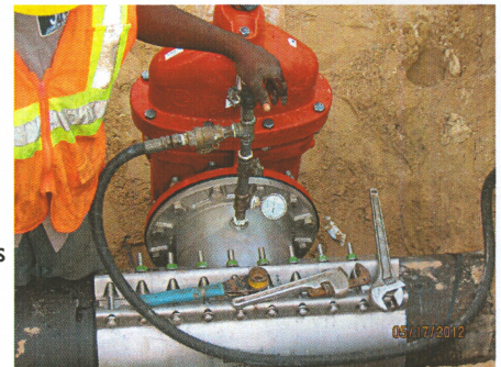
Tapping sleeve and valve are pressure tested prior to performing wet tap.
