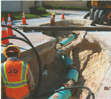
Jeff Brady's crew snakes new 18 inch force main over, under, and around the many conflicts in Ocean Avenue.
