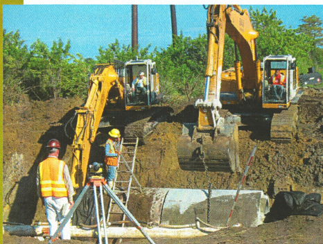
St Lucie County Shinn Road Emergency Repair: David Reid's crew placing 84 inch RCP. Work commenced two days after the project was bid and awarded. The area had to be open to emergency traffic within five days and completed within five more days. Four crews worked 12 hour shifts through the night to successfully meet this deadline.
