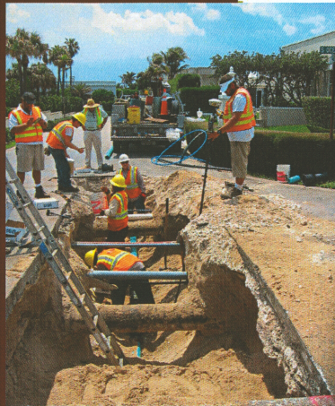
Surveyor and inspector record the location of the numerous existing utility pipes in Ocean Avenue.
