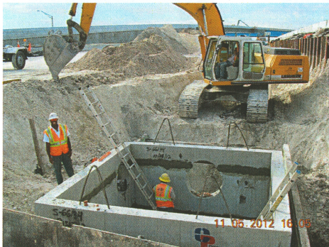
I-595: Stern Lashley and crew installing another weir control structure as part of the I-595 Express Segment C project for Bergeron Land Development.
