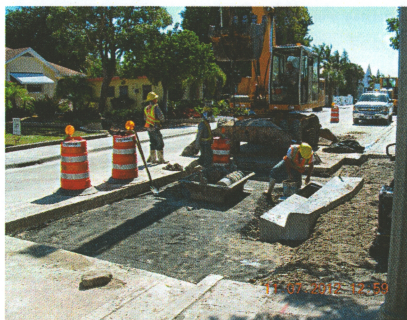
FDOT District 4 Drainage: Jeff Brady and crew making drainage improvements on Federal Highway in Lake Worth as part of our contract.
