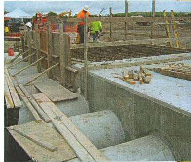
In progress installation of storm water structure (staging shown far left).
