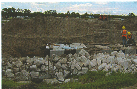
Renel Louisca and Erick Bagford work on installation of 10x3 box culvert.
