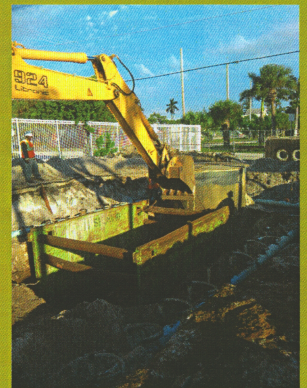
Riviera Beach Marina: Chesca Ceance's crew preparing to tie 8 inch gravity sewer into lift stations for the City of Riviera Beach.
