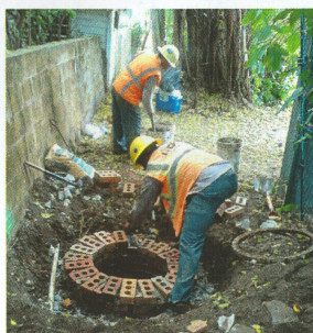
Town of Palm Beach Sewer/Storm Rehabilitation: Odi Hernandez and crew replaced 8 inch sewer main in an alleyway at Brazilian using only a mini and hand digging due to space constraints (above and right).
