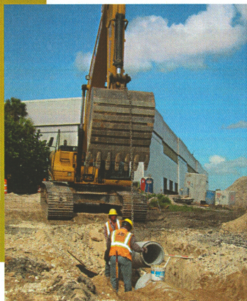
Larry Heffner and Renel Louisca install 24 inch RCP up to the tipping floor of the recycling building.
