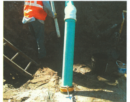
10th Street in Ft Pierce: Tom Linsley's crew installing a 6 inch saddle and service pipe on lined 30 inch clay sewer pipe for Dickerson Florida Inc.
