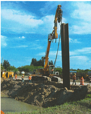
I-595: Stern Lashley and crew installing another weir control structure as part of the I-595 Express Segment C project for Bergeron Land Development.
