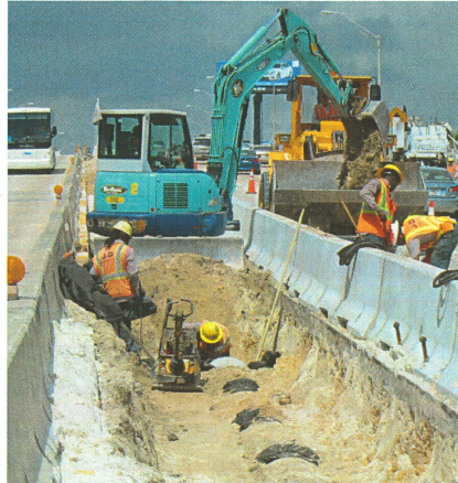
SR-112: Odi Hernandez's crew installing 18 inch RCP in the median for Condotte America. The median was less than 10 feet wide and provided just enough room for a mini to operate. The loader transported each individual piece of pipe to the crew when the crew was ready to install it.
