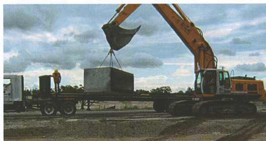
Pipelayer Larry Heffner and Backhoe Operator Kevin Maag taking delivery of 10x3 box culvert.
