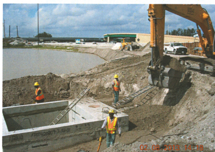
I-595 Segment E: Stern Lashley and crew installing a control structure at Florida's Turnpike for Ranger Construction and Dragados.
