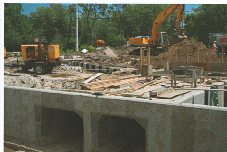
Sarno Lakes: (Left) Jeff Brady and crew support a 20 inch prestressed concrete water main in advance of installation of twin 8x4 box culverts for Brevard County. (Right) Mosley & Son Construction poured a junction box to tie together the three way box culverts (6x5, 7x5, and 7x5) installed by Dave Reid's crew.
