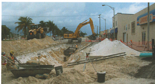
Old Pompano Water and Sewer: Chescal Ceanse's crew installing deep sewer for Burkhardt Construction.
