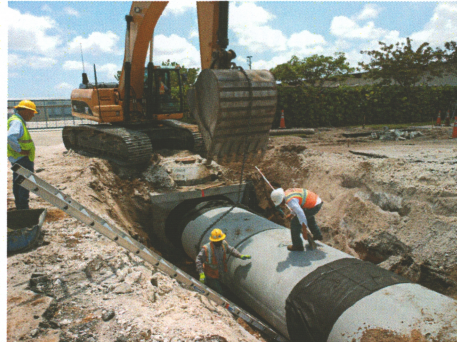
Clark Cryer and crew installing 43x68 into a manhole.
