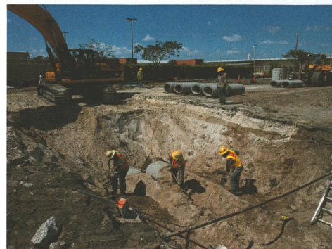
Clark Cryer's crew installing double barrel 19x30s.
