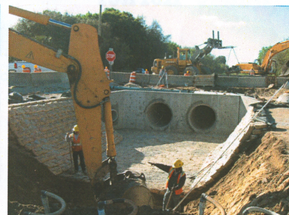
Orange Avenue: (Left) JJ Williamson's crew setting double barrel 60 inch RCP in canal 56 for St Lucie County. (Right) Over 3,600 individual bags of sand cement riprap were placed at the base and along the sides of the canal for canal bank stabilization.
