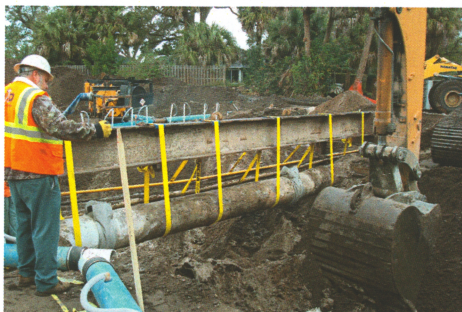
Sarno Lakes: (Left) Jeff Brady and crew support a 20 inch prestressed concrete water main in advance of installation of twin 8x4 box culverts for Brevard County. (Right) Mosley & Son Construction poured a junction box to tie together the three way box culverts (6x5, 7x5, and 7x5) installed by Dave Reid's crew.
