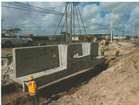
Chescal Ceance's crew setting a double barrel 19x30 headwall/control structure.
