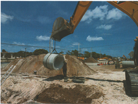
Backhoe Operator Kevin Maag and Skilled Laborer Charles Simms prepare to install the cut piece into the structure as three other J-D crews work in the background.
