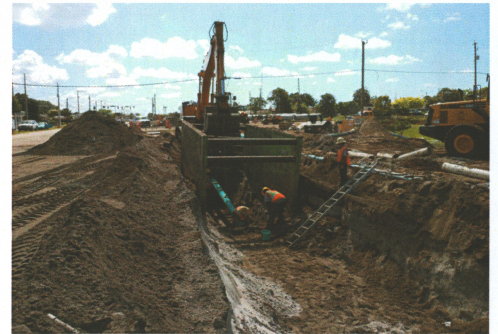
Odi Hernandez and crew installing 10 inch sanitary sewer.
