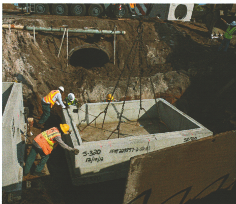
Chescal Ceance and crew setting 58x91 conflict structure for 24 inch double barrel drainage.
