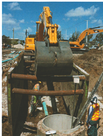
Chescal Ceance's crew installing 8 inch sanitary sewer.
