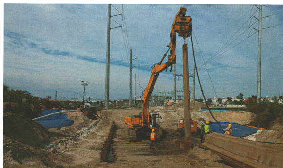
FPL 24 inch pipeline: JJ Williamson and crew sheeting and dewatering for Troy Construction for a 140 foot offset under a canal.
