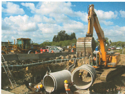
Orange Avenue: (Left) JJ Williamson's crew setting double barrel 60 inch RCP in canal 56 for St Lucie County. (Right) Over 3,600 individual bags of sand cement riprap were placed at the base and along the sides of the canal for canal bank stabilization.
