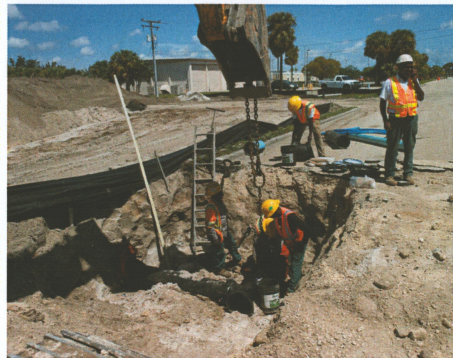
JJ Williamson and crew installing water main.
