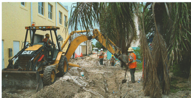
Old Pompano Water and Sewer: Sergio D. Filipone and crew install water and sewer services in an alleyway for Burkhardt Construction.
