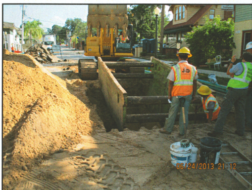
Gravity sewer pipe being installed on Alexander Street.
