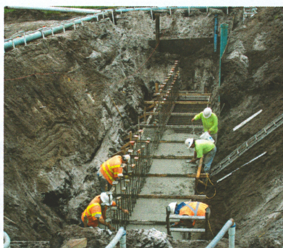
SE Heritage Ridge Boulevard: After Tom Linsley's crew dewatered and excavated a 18 foot cut for J.W. Cheatham and Martin County Engineering, our subcontractor Mosley & Son Construction began work on the footer for a 84 inch headwall.
