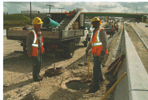
I595 Segment E: Tony Estep and Aniel Phanor working on one of the many manhole and barrier wall inlet adjustments for Ranger Construction.
