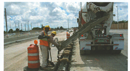
I 595 Segment E: Everton Henry and Agustin Guerrero Oseguera handled all construction components for the trench drain installation including saw cutting, excavation, panel installation, and final concrete pour for Ranger Construction.
