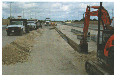
I 595 Segment E: Everton Henry and Agustin Guerrero Oseguera handled all construction components for the trench drain installation including saw cutting, excavation, panel installation, and final concrete pour for Ranger Construction.
