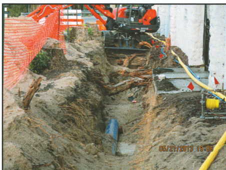
Watermain installation on 5th Avenue, looking west.
