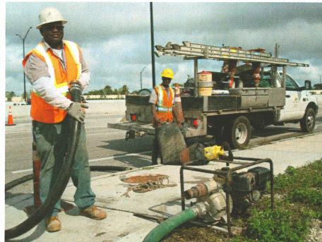
I595 Segment C: Jerry Davis and Kenny Harp work through extensive drainage system finals for Bergeron Land Development including using airbags for pumping down systems while contending with traffic and other hurdles.
