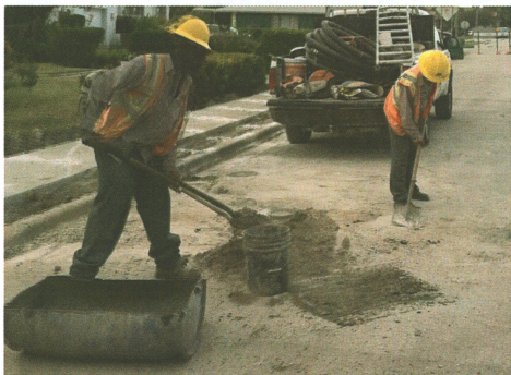
SR 710 Riviera Beach: Lenny Arce Urieta and crew adjust valve boxes for the final lift of asphalt after installation of new watermain for Ranger Construction.
