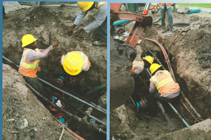
Town of Palm Beach Ejector Station Upgrade: Chesca Ceance's crew is tying in our newly installed forcemain to a lift station for Murray Logan Construction.
