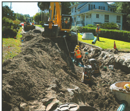
Sanitary sewer pipe installation on 3rd Avenue.
