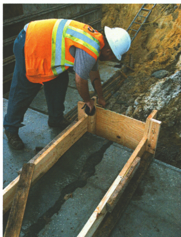
Lakewood Park Canal: Form work to connect to new box culvert being installed by Richard Tharpe and crew for St Lucie County.
