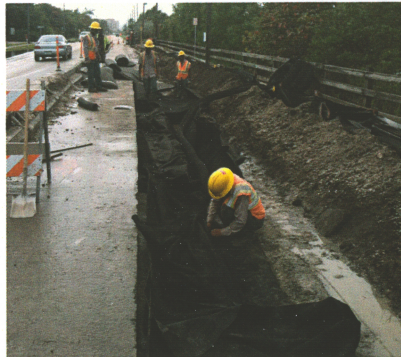
SR A1A: Lenny Arce Urieta and crew install edge drain for Weekley Asphalt Paving.
