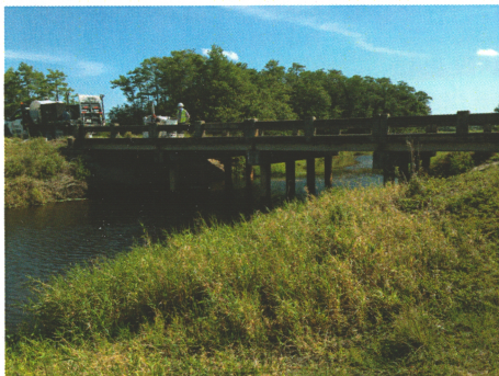
CR 708: (Left) ABC Concrete Cutting getting ready to saw cut the existing bridge deck for removal of the bridge. (Right) Tom Linsley and crew backfill the segmental bridge after installation. The project is being constructed for J.W. Cheatham, LLC and Martin County.
