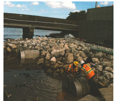
Flagler Memorial Bridge: Odi Hernandez and crew install 36 inch and 48 inch RCP and flap gates for PCL Constructors.
