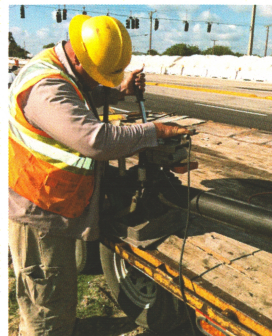
Phil McDonald fuses 4 inch HDPE for the directional bores on the US1 crossing.
