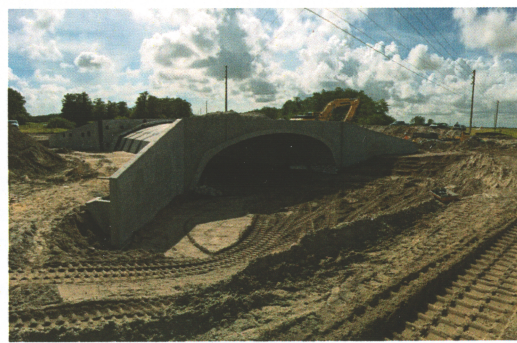
CR 708: (Left) ABC Concrete Cutting getting ready to saw cut the existing bridge deck for removal of the bridge. (Right) Tom Linsley and crew backfill the segmental bridge after installation. The project is being constructed for J.W. Cheatham, LLC and Martin County.
