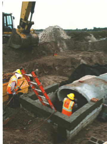
North County Aviation Wetlands Mitigation: Dave Fayssoux's crew does mud work for 34x53 pipe for Rio-Back Corporation and Palm Beach County.
