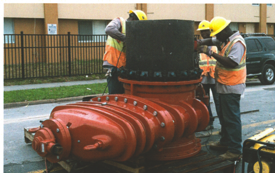
Flagler Memorial Bridge: Odi Hernandez and crew install 36 inch and 48 inch RCP and flap gates for PCL Constructors.
