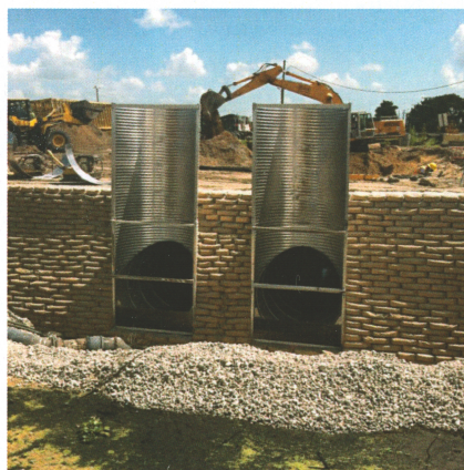
Osceola Sugar Mill: Odi Hernandez and crew installed double barrel 72 inch sand cement rip rap headwall with two 72 inch flashboard risers. The sand cement was hand placed by for Rio-Bak Corporation.
