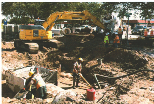
SR70: Pipelayer Mateo Torres Mendez and Tailman Andres Pascual on Jeff Brady's crew backfill and compact around an inlet for Ranger Construction.
