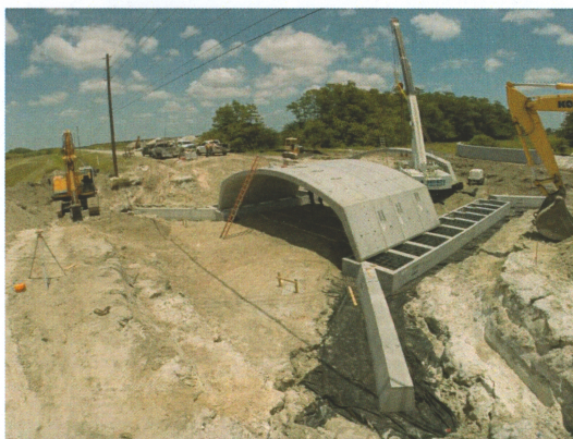
CR 708: Tom Linsley and crew set nine segments of a 40 foot span, 10 foot rise CON/SPAN for JW Cheatham.
