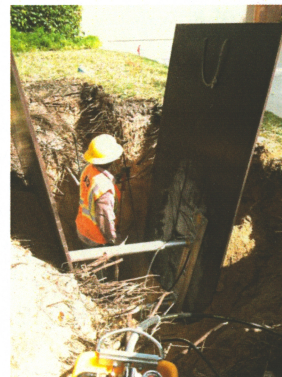
Jupiter Bluffs/ Jupiter Utility Repairs and Improvements: Dan Follett and crew installing new water taps for the Town of Jupiter.
