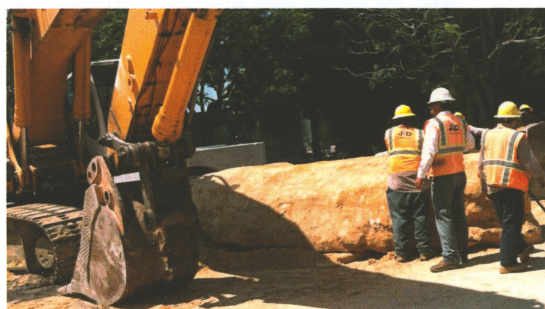
SR 5 Cocoa: Tom Linsley and crew working for Astaldi Construction unexpectedly ran into a large shelf of hard rock that required the use of a Backhoe-mounted hammer to break prior to removal by the 954 with its rock bucket.
