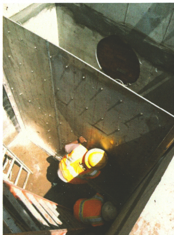
St Vincent de Paul Regional Seminary: Everton Henry and crew installs a weir control structure for CSR Heavy Construction.
