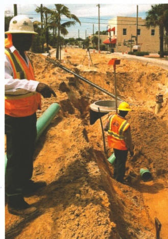
Installing sanitary sewer.
