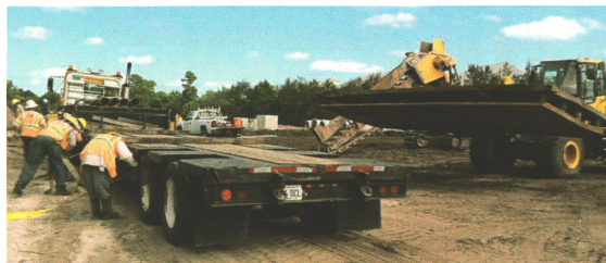
Odi Hernandez's crew including Loader Operator Gordon Davio unload a trench box delivered by Truck Driver Bob Parkinson. They will need the trench box for pipe and structure installation near the roadway 10 feet deep.
