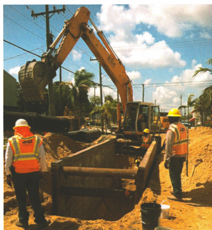
Installation of 30 inch water main.
