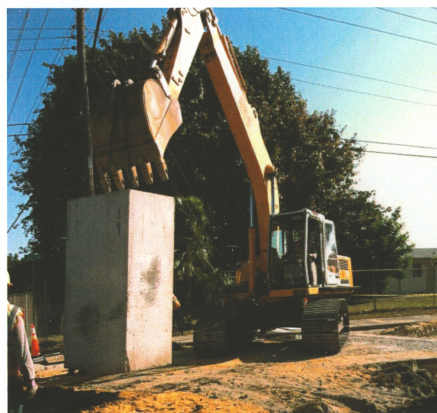
Dave Fayssoux's crew installing drainage.
