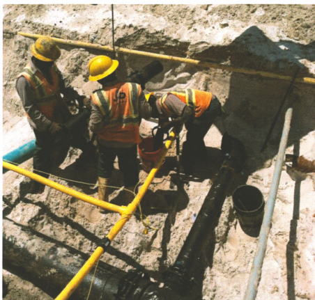
Chescal Ceance's crew making a tie in on a 16 inch to 6 inch water main.
