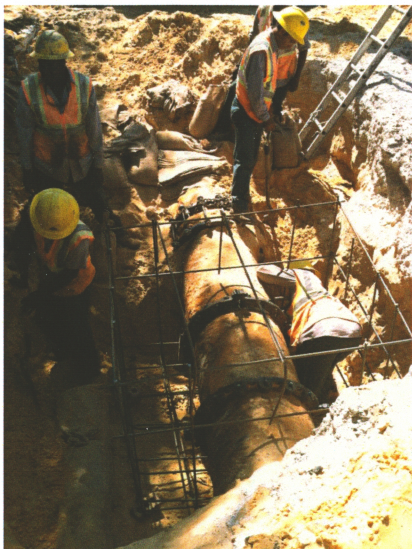
Chescal Ceance's crew installing a thrust collar for a 24 inch gate valve.
