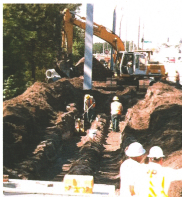
Pablo Fernandez Vargas and crew install 24 inch pipe. The backhoe had to dig between two power poles.
