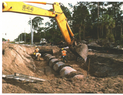
Installation of 24 inch RCP.
