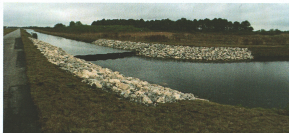
SR 70/FDOT Push-Button Contract: Jeff Brady and crew installed rock rubble for bank protection for two steel sheeting weirs that had been washing out prior to repairs. The existing sheet pile was extended between 10 to 12 feet into the banks, and approximately 800 tons of bank and shore rip rap material were installed for bank stabilization between the two locations.
