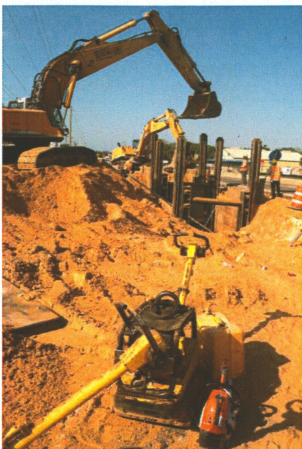
SR 5 Cocoa/Astaldi Construction: (Left) David Reid's crew assembles a slide rail system. (Right) The crew installed 48 inch pipe in depths up to 20 feet using this system. After compaction the crew removed the panels as they back-filled and repeated the process for 1,000 feet.
