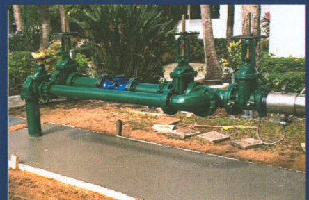
Jupiter Utility Repair/Town of Jupiter: Lenny Arce Urieta and crew took the below meter assembly and raised it above ground. The crew did all associated work including the concrete.
