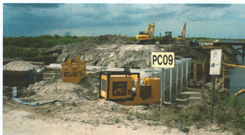
PC09 Culvert Replacement/Rio-Bak Corporation: Pablo Fernandez Vargas and crew held the Miami Canal back while installing five barrel 84 inch culvert.
