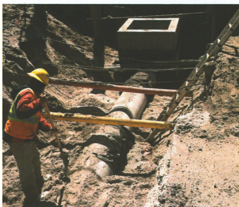
Pipelayer Santos Arce installs drainage under existing utilities.
