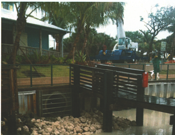
Jerry Philbrick and crew install rubble rock in front of existing 42 inch outfall.
