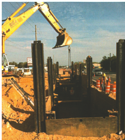
SR 5 Cocoa/Astaldi Construction: (Left) David Reid's crew assembles a slide rail system. (Right) The crew installed 48 inch pipe in depths up to 20 feet using this system. After compaction the crew removed the panels as they back-filled and repeated the process for 1,000 feet.
