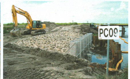
PC09 Culvert Replacement/Rio-Bak Corporation: Pablo Fernandez Vargas and crew held the Miami Canal back while installing five barrel 84 inch culvert.
