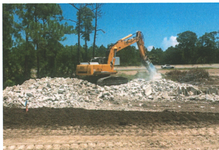
I95 SR 512 to Brevard County Line: David Reid and crew crushed Community Asphalt's existing barrier wall and box culverts that were to be replaced. The material was recycled into bedding stone for the new culverts.
