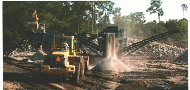
I95 SR 512 to Brevard County Line: David Reid and crew crushed Community Asphalt's existing barrier wall and box culverts that were to be replaced. The material was recycled into bedding stone for the new culverts.
