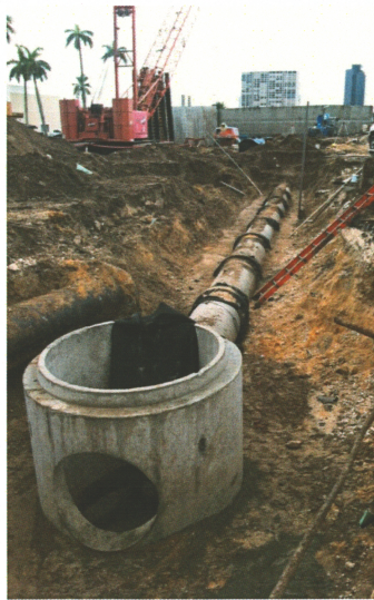
Installation of 30 inch drainage.
