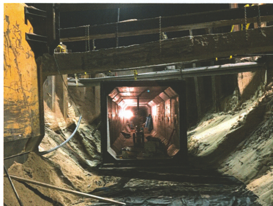
Installation of culvert under existing utilities.
