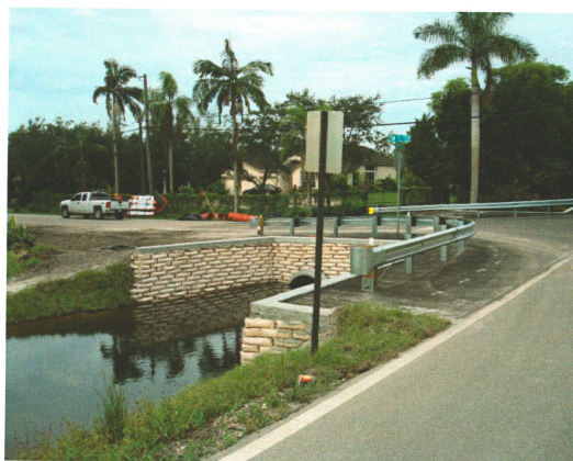
S-24 Culvert Replacement: Chesca Ceance's crew installed double barrel 54s including the hand-forming of sand cement rip rap walls to allow the widening of 111th Terrace, within the Central Broward Water Control District canal right of way.
