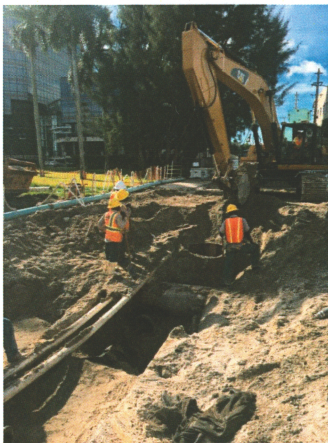
Chescal Ceance and crew installing 18 inch gravity sewer.
