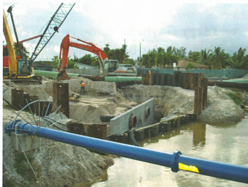
City of Sunrise Pump Station 2 Outfall: Odi Hernandez's crew installed two 36 inch DIP and one 60 inch RCP for Murray Logan Construction.
