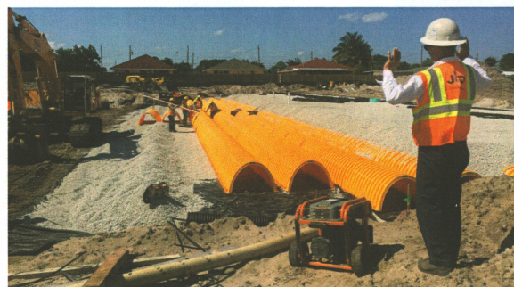
2773 Public Charter School: Norm Weaver guides Jerry Philbrick's crew installing a Storm Tech drainage system for Hardrives. This system is installed beneath a parking lot and eliminates the need for an onsite retention pond.
