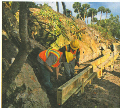
Jamie Camargo and Luis Ruiz measure and cut forms around the cap rock.
