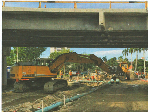
Flagler Memorial Bridge: Jerry Philbrick's crew lays 18 inch gravity sewer under the Flagler Bridge for PCL Constructors.
