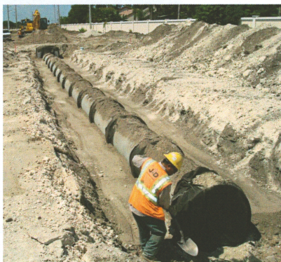
Hiatus Road: Pipelayer Tranquilino Velasquez installs a 36 inch drainage trunkline for Marks Brothers.
