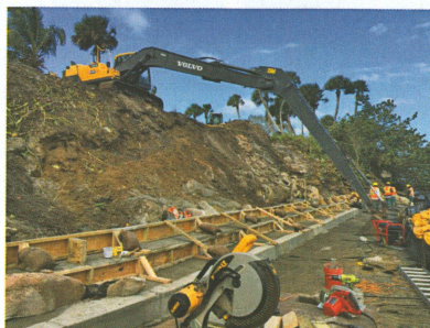
Forming up before pouring flowable fill into the voids of the cap rock.
