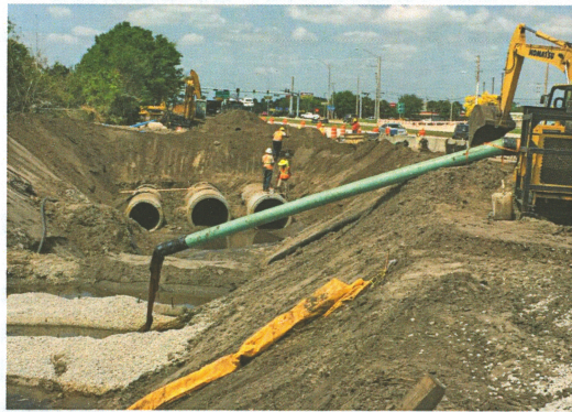
SR 70: Tom Linsley and his crew lay 60 inch and 48 inch RCP in a canal for Ranger Construction.
