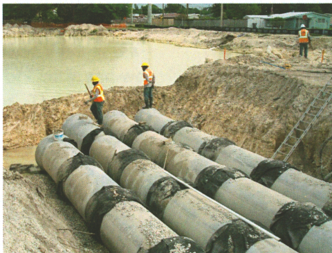
SR 7: Dave Fayssoux's crew installs 36 inch quad RCP connecting to drainage ponds for Community Asphalt.
