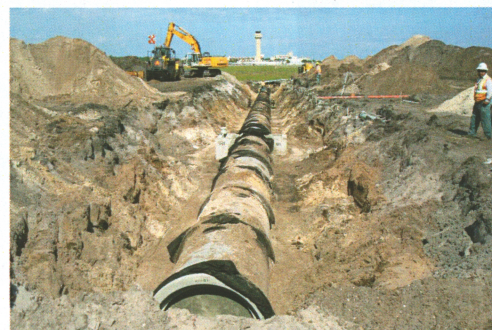
PBIA Taxiway W: Odi Hernandez and crew install 48 inch RCP crossdrain for Rosso Site Development.
