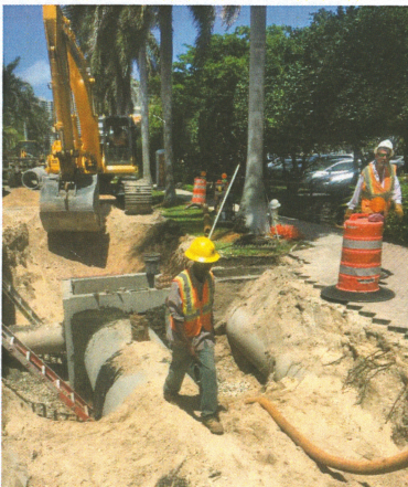
Ocean Avenue Drainage Improvement: Dave Fayssoux and crew install a 42 inch drainage manhole for the Town of Palm Beach Shores.
