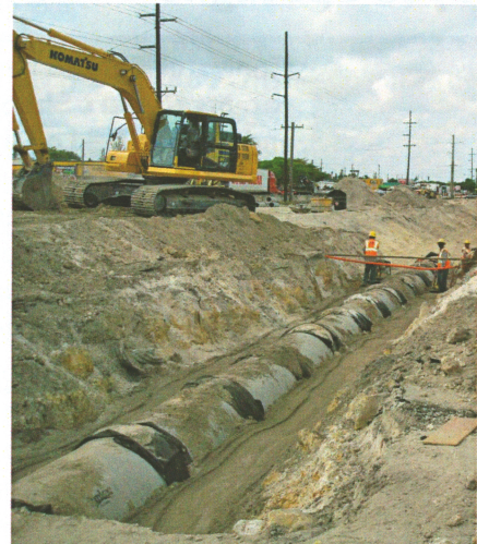
SR 7: Odi Hernandez's crew installs 42 inch side drain culvert for Community Asphalt.
