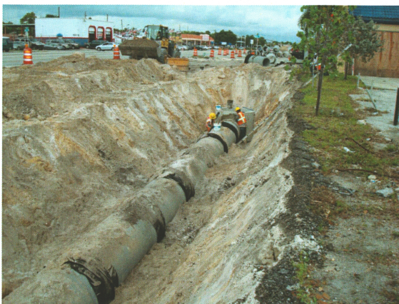
Stern Lashley and crew install a 42 inch trunkline.
