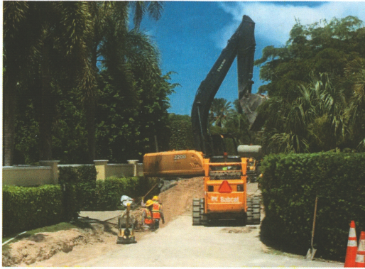
Crew installing drainage on Cherry Lane working in limited workspace due to existing utilities and private landscaping.
