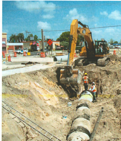
Stern Lashley and crew lay 36 inch concrete pipe.
