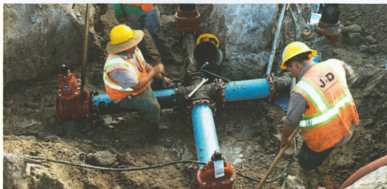
Rene Hernandez crew assembling a watermain intersection located at Appaloosa Trail and Equestrian Way.
