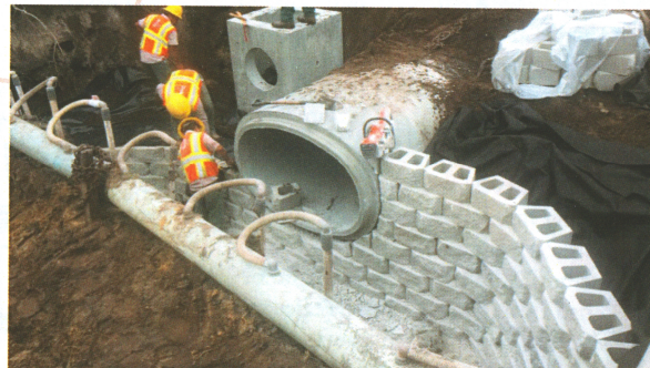
Emergency Culvert Replacement 33rd Avenue at 16th Street: Left: Road washed out prior to Johnson-Davis work. Center: Jeff Brady and crew install new culvert and articulated block wall in lieu of alternate approaches to help with community beautification. Right: Final product for the City of Vero Beach.
