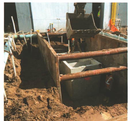
Healthy Living Grease Traps: Jacky Henrisme and crew install the first of three grease traps for Medic Air Systems.
