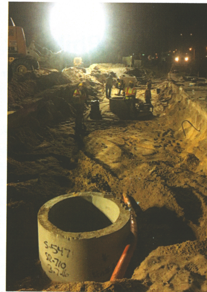
SR 710 T4418: Sergio D Filipone's crew installing 18" pipe across Australian Avenue at night for JW Cheatham.
