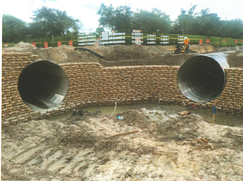
B Road: Chescal Ceance's crew removed two bridges and installed 96" CAP pipe and headwall with wings for Hardrives of Delray.
