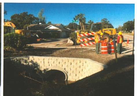
Emergency Culvert Replacement 33rd Avenue at 16th Street: Left: Road washed out prior to Johnson-Davis work. Center: Jeff Brady and crew install new culvert and articulated block wall in lieu of alternate approaches to help with community beautification. Right: Final product for the City of Vero Beach.
