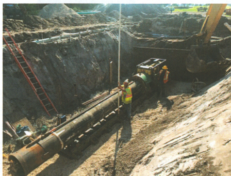
Beaumont Avenue: Central Florida Underground does a jack and bore under the railroad tracks on Beaumont Avenue. David Richards and crew excavated the trench for Burkhardt Construction and also assisted setting up the bore operation.
