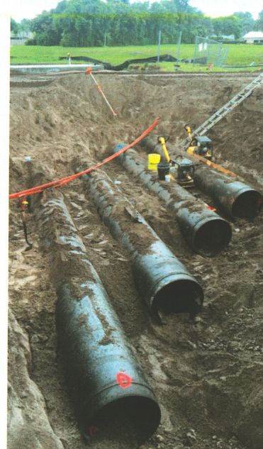
C-17 30" Crossing: Installed four 30" DIP for C-17 Pump Station crossing Congress Avenue for Murray Logan Construction.
