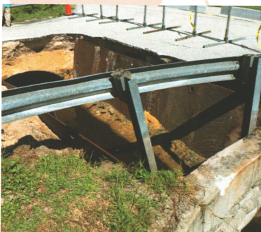
Emergency Culvert Replacement 33rd Avenue at 16th Street: Left: Road washed out prior to Johnson-Davis work. Center: Jeff Brady and crew install new culvert and articulated block wall in lieu of alternate approaches to help with community beautification. Right: Final product for the City of Vero Beach.
