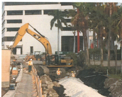
Flagler Memorial Bridge: Foreman Odi Hernandez keeps a watchful eye from the bridge deck as his crew installs 30" French drain for PCL Constructors.
