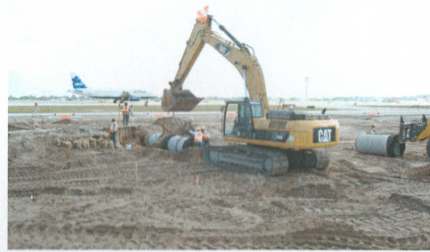
PBI Runway 10R-28L Rehabilitation: Odi Hernandez's crew extend a 36" outfall for Ranger Construction.
