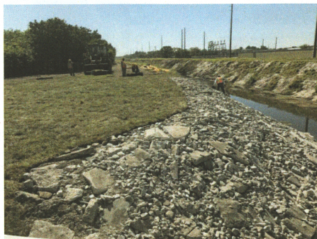
27th Avenue Headwall Outfall Replacement: Aristhene Thelisonort's crew was responsible for the complete 66" outfall installation for the City of Vero Beach. The work included removing a 66" headwall and then reinstalling 66" pipe, rock rubble, and sod.
