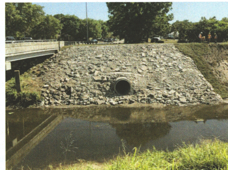
27th Avenue Headwall Outfall Replacement: Aristhene Thelisonort's crew was responsible for the complete 66" outfall installation for the City of Vero Beach. The work included removing a 66" headwall and then reinstalling 66" pipe, rock rubble, and sod.
