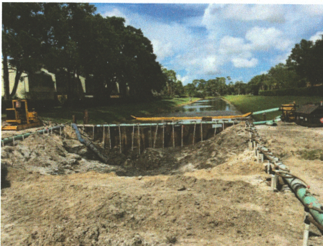
Big Blue Trace: Cofferdam installation and 72 inch storm drain installation as part of the Village of Wellington's road restoration project.
