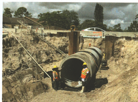
Big Blue Trace: Cofferdam installation and 72 inch storm drain installation as part of the Village of Wellington's road restoration project.
