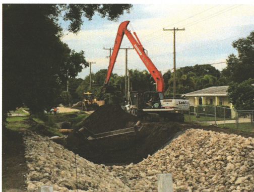
Dirt out, filter fabric, bedding stone, and riprap in.
