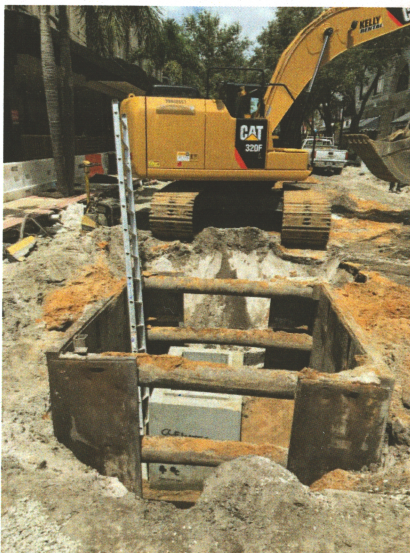
Clematis Streetscape: Odi Hernandez and crew installing drainage and watermain in the heart of downtown as part of Burkhardt Construction's beautification project for the City of West Palm Beach.
