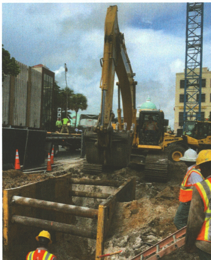
Former City Hall- Woodfield Apartments: Chescal Ceance and crew installing the exfiltration storm drainage for American Engineering & Development.
