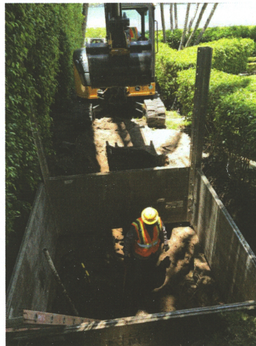
Palm Beach Private Residence: Sergio D. Filipone's crew excavating for a doghouse sewer manhole as part of a sewer renovation for Hedrick Brothers Construction.
