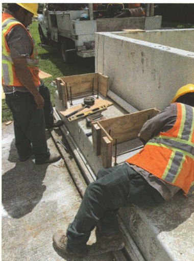
Lyons Road Force Main north of Palmetto Park Road: (Left) Humberto Gil Vazquez builds a pier for an aerial crossing for Palm Beach County Water Utilities Department. (Right) Chesal Ceance and crew install the 12 inch force main aerial.
