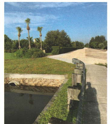
N-29A Canal Connector: After Odi Hernandez's crew installed 72 inch drainage, Gene Hayford's crew performed restoration including constructing a TRUEGRID fire access road for the Central Broward Water Control District.
