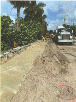
Flowable fill was used to protect the double barrel 12" drainage pipes
