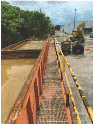
Riverwalk: James Albritton's crew uses a weir tank to dewater in order to reduce turbidity, prior to 10 foot sewer installation for American Engineering and Development.
