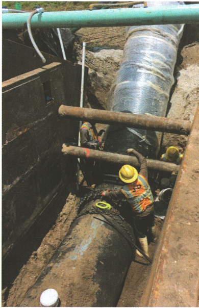
Atlantic Avenue and the Turnpike: (Left) Jacky Henrisme's crew installs 42 inch watermain. (Below) Completed aerial crossing of the watermain for Ranger Construction Industries.
