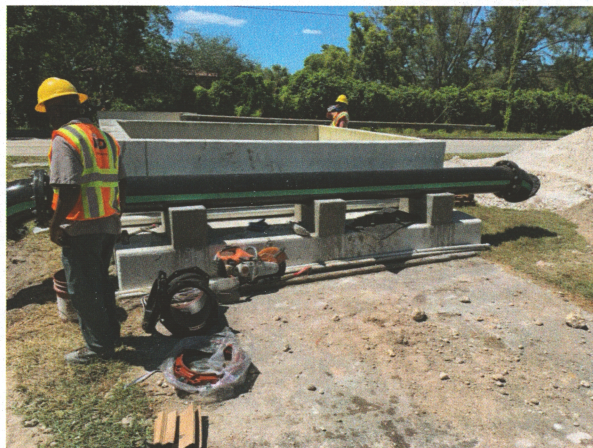
Lyons Road Force Main north of Palmetto Park Road: (Left) Humberto Gil Vazquez builds a pier for an aerial crossing for Palm Beach County Water Utilities Department. (Right) Chesal Ceance and crew install the 12 inch force main aerial.
