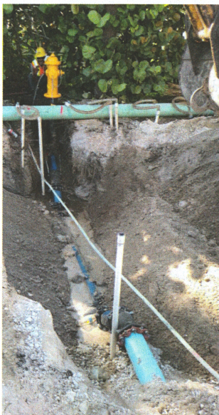
Crew installing 6" watermain deflection to the new fire hydrant prior to installation of the new drainage
