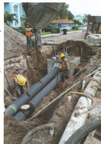
Crew installing double barrel 12" drain line on South Lakeside Drive
