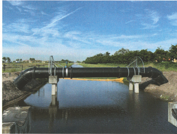
Atlantic Avenue and the Turnpike: (Left) Jacky Henrisme's crew installs 42 inch watermain. (Below) Completed aerial crossing of the watermain for Ranger Construction Industries.
