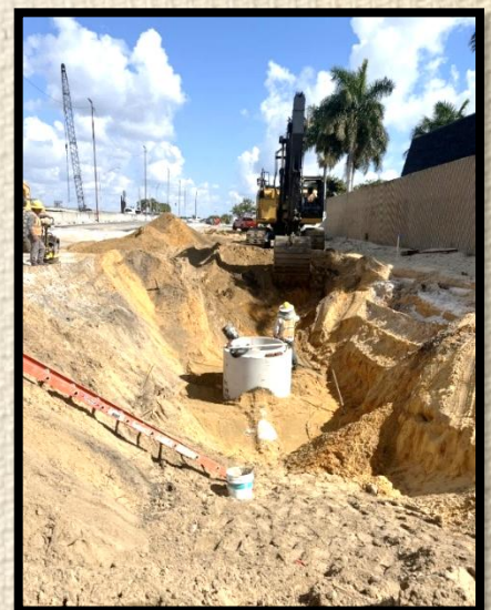
Pictured above: Installation of various storm drainage systems on the off ramp of I-95 adjacent to Boynton Beach Boulevard.
