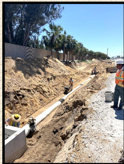
Pictured above: Installation of various storm drainage systems on the off ramp of I-95 adjacent to Boynton Beach Boulevard.
