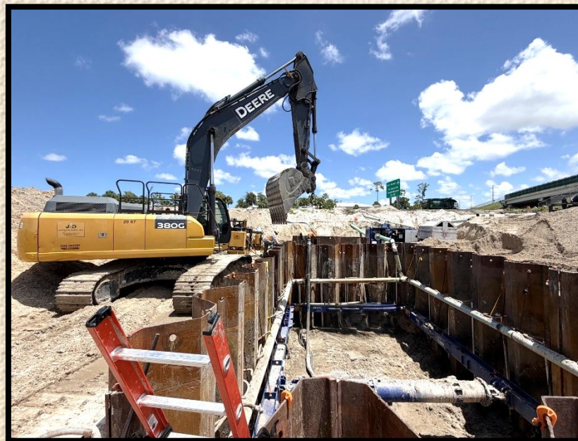
Pictured above: Installation of a jacking pit for micro tunneling. A 51" casing under the turnpike will then house a 30" watermain. Joe Bagford, Superintendent; Pablo Fernandez, Foreman
