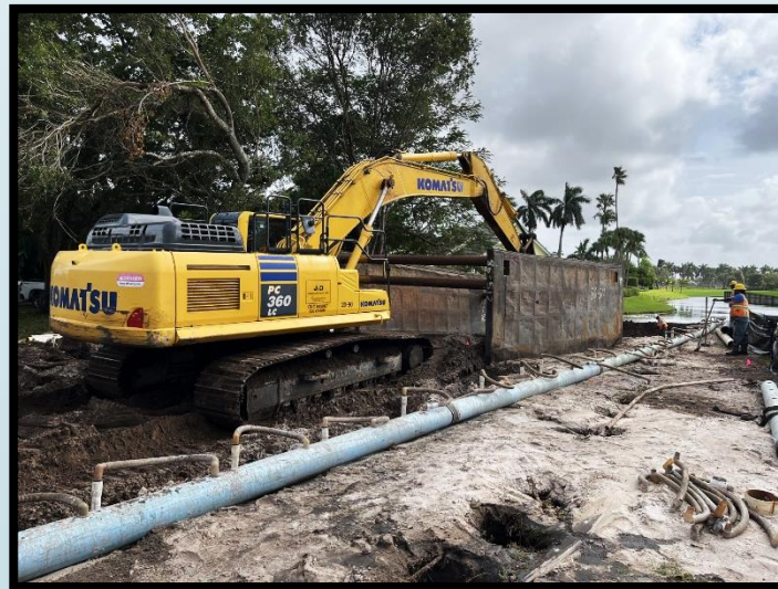
Above: Replacement of existing drainage control structure and outfall at St. Andrews Country Club. Stern Lashley, Foreman; Joe Bagford, Superintendent
