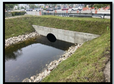
Above left to right: Progression of converting an existing bridge into a culvert
