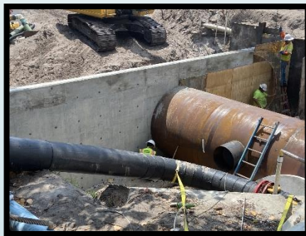
Above left to right: Progression of converting an existing bridge into a culvert
