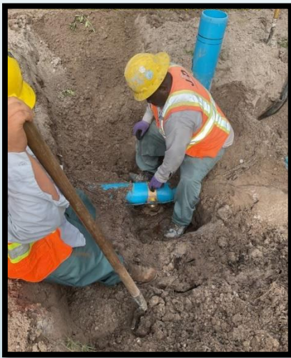
Water service tap for new 6" watermain
