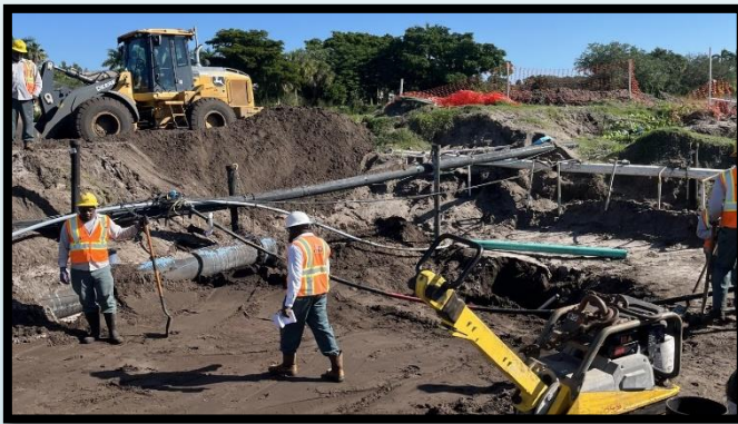
Pictured above: Chescal Ceance (foreman) supervising the installation of 18" watermain
