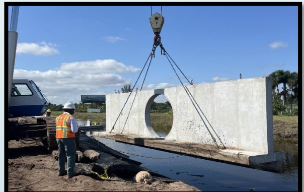
Pictured above: Wisler Dort (foreman) supervising the installation of 60" concrete endwall
