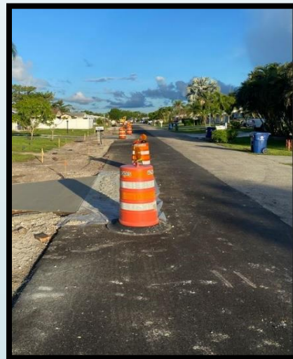
Final resurface of new drainage
