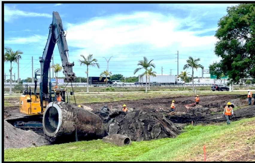
Above: Demolition of existing drainage system at Boca Airport service road in preparation of installation of new stormtech drainage system. Walt Pfaffenberger (PM), Joe Bagford (Superintendent), Joe Johnson (Foreman)
