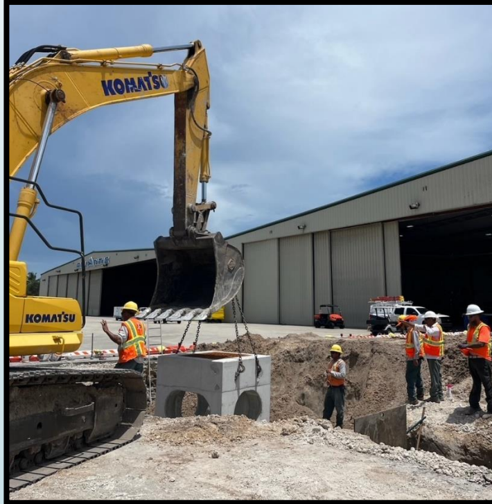
Pictured above: Setting concrete drainage structure at Atlantic Aviation. Walter Pfaffenberger (Project Manager), Leonard Dennis (Superintendent), Jeff Brady (Foreman)
